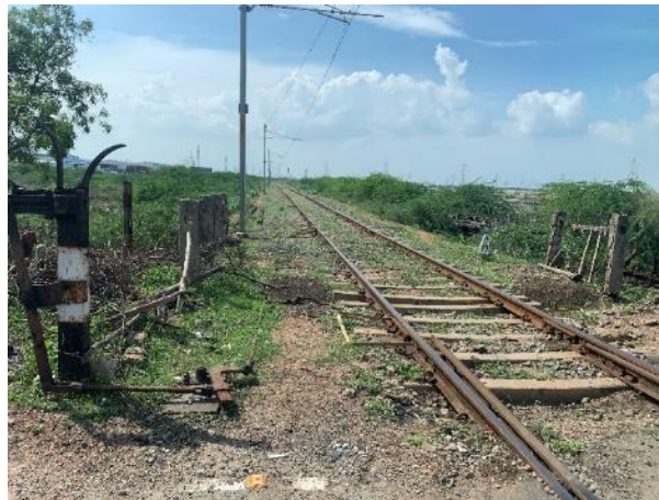
Railway connectivity at Port
