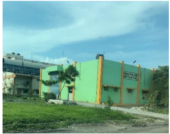
View of the 22 kV Centralized Electrical Control Room within VOC Port
