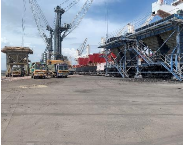
View of the Equipment located within Berth 9
