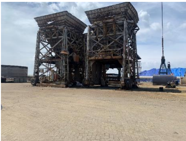
View of the Equipment located within Berth 9
