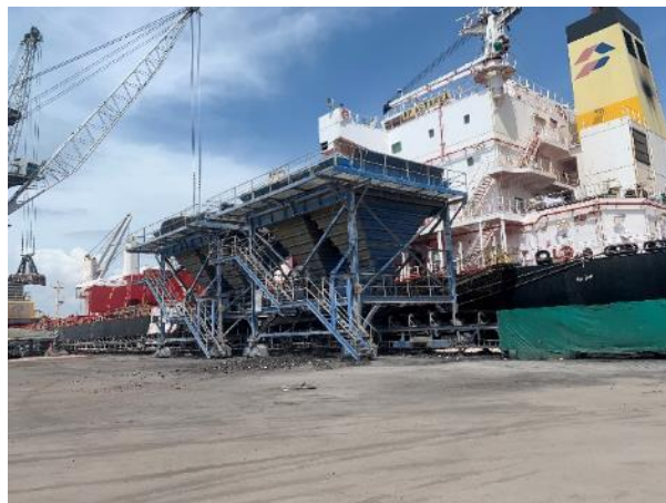
View of unloading activity performed at Berth 9 by existing terminal contractors
