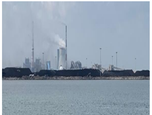
Long View of the Coal Stackyard located towards the Northwestern direction of Berth 9
